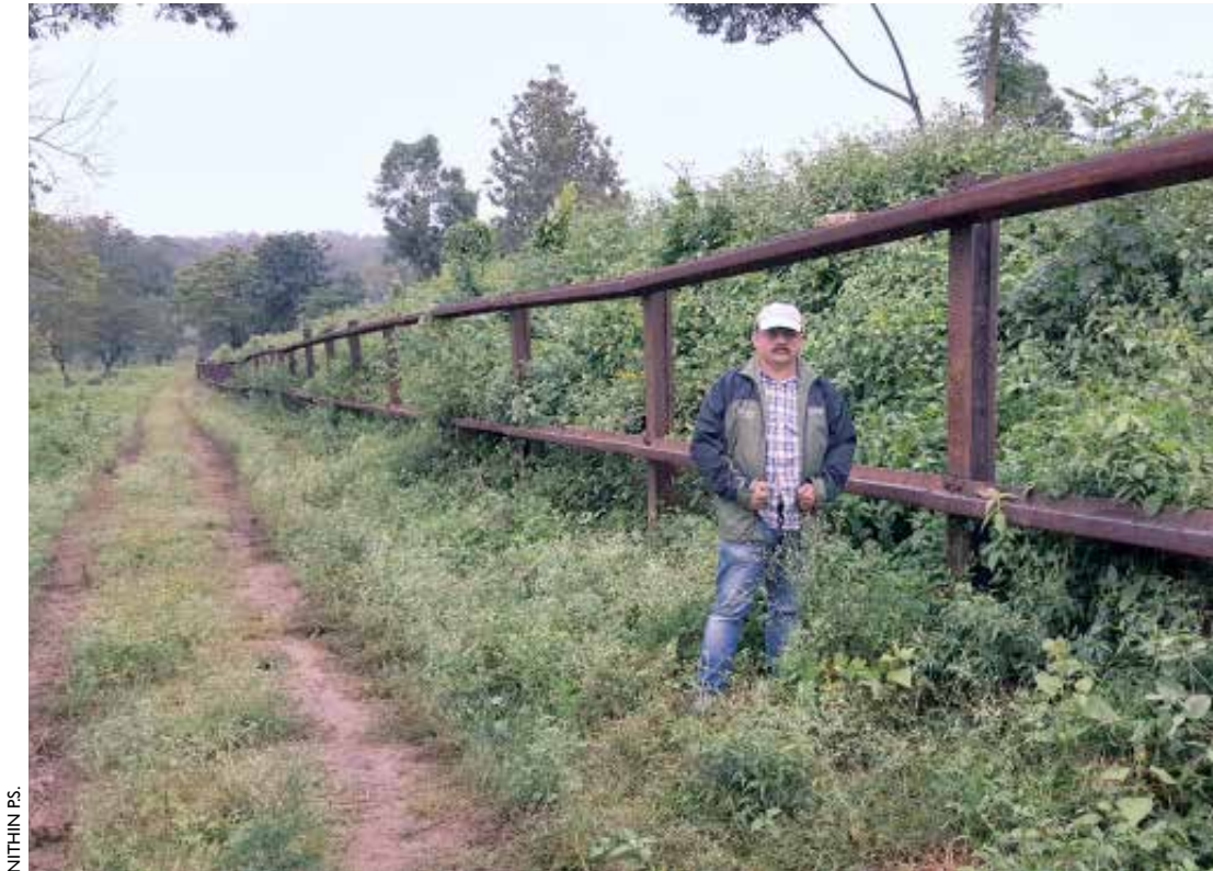
Rail fence at Nagarhole NP, (note the height of fence is only about 2 m)
