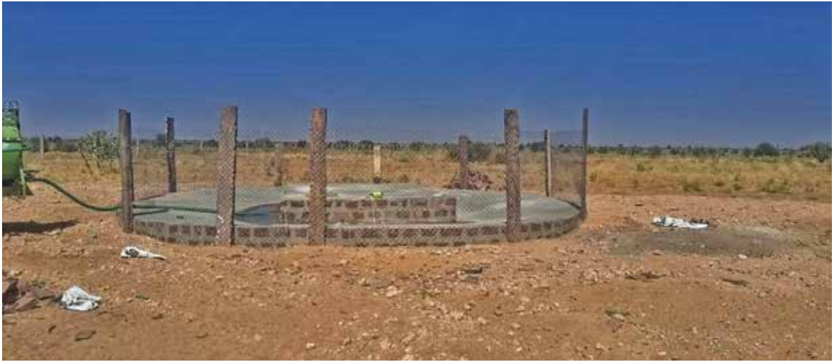
An underground storage tank has been constructed on BNHS land as part of the initial infrastructure development for the field research station
