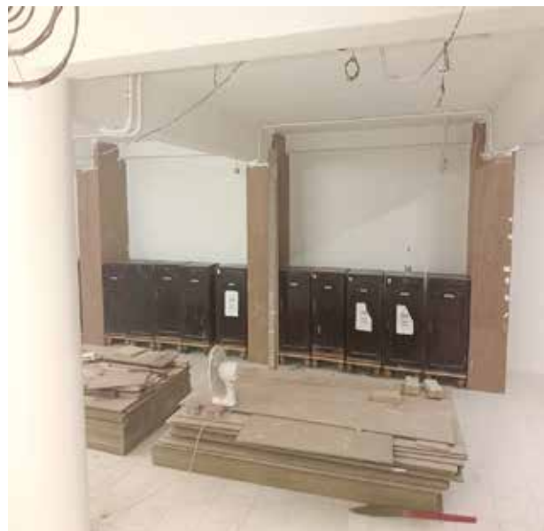
Wooden partition for corners and stairs have been installed on the mezzanine floor
