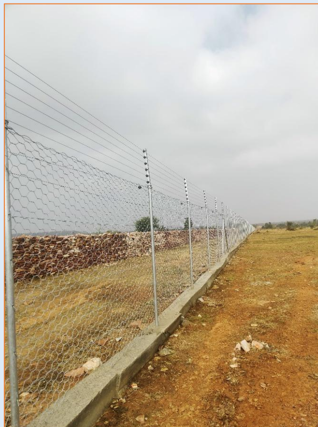
Predator-proof fencing is being developed for the Cheetah Reintroduction Program in the Gandhi Sagar Wildlife Sanctuary, Madhya Pradesh © Sujit Narwade
